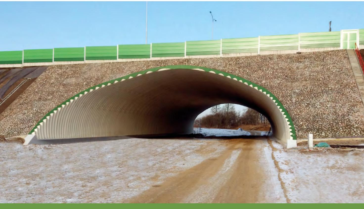
” UltraCor® versatile structures are used for roads, railways and industrial applications as well as for reinforcement and reconstruction of existing structures such as:
